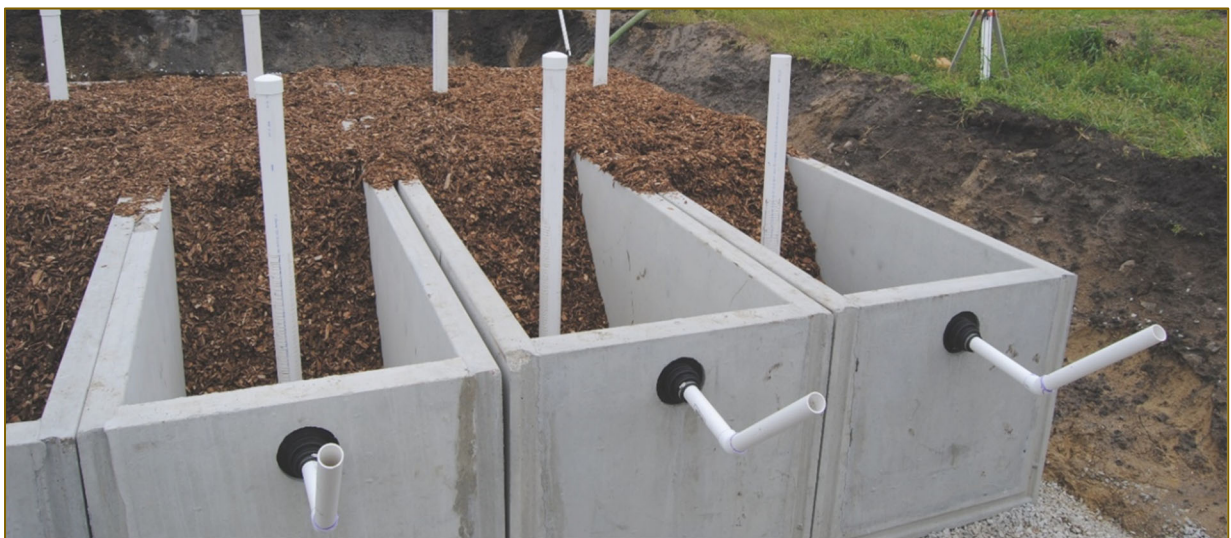
Image: Bioreactor used to decrease nitrate-nitrogen being deposited in waterways
